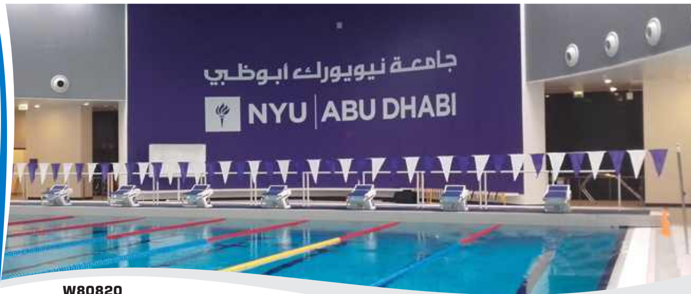
W80820 Movable Bulkhead
